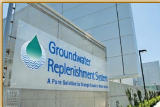
▲ Recycle wastewater to raise its productivity, as this sewage treatment plant does for Orange County, California.
